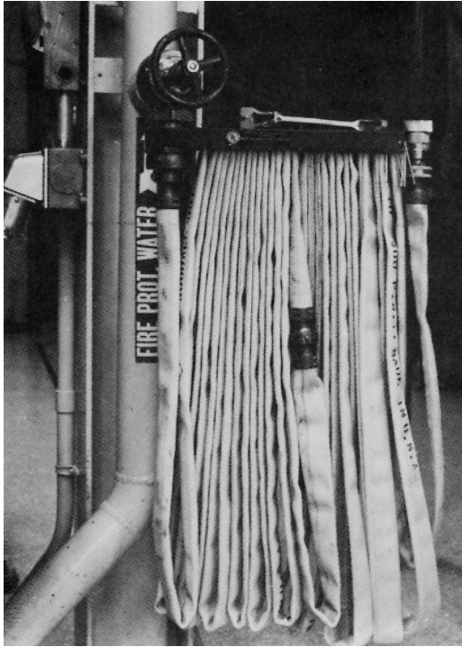
FIGURE A.3.3.19.1 Conventional Pin Rack.
