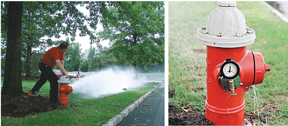
Exhibit 21 Flushing of Residual Hydrant (left) and Attachment of Test Equipment (right).
