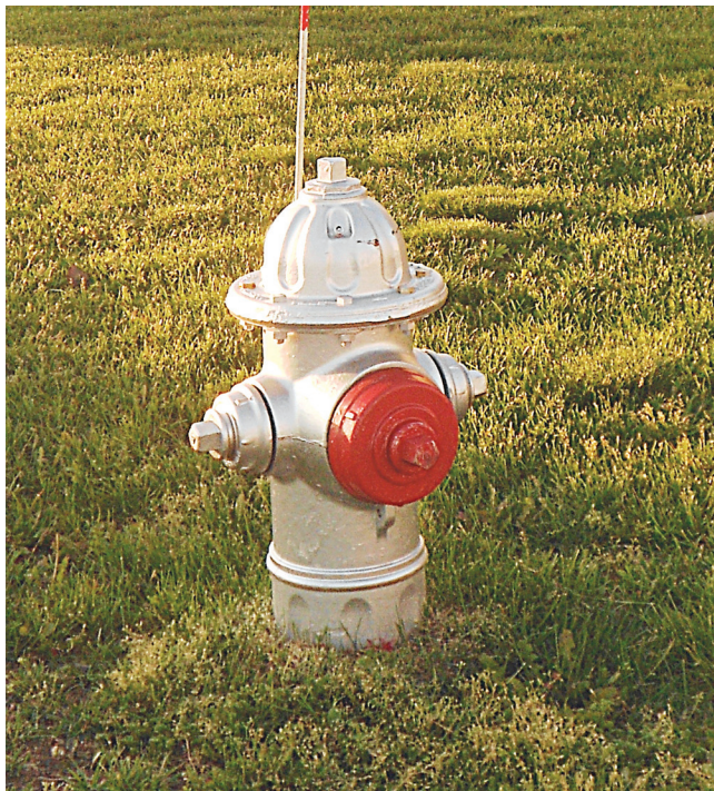
EXHIBIT 2 Dry Barrel Hydrant.
