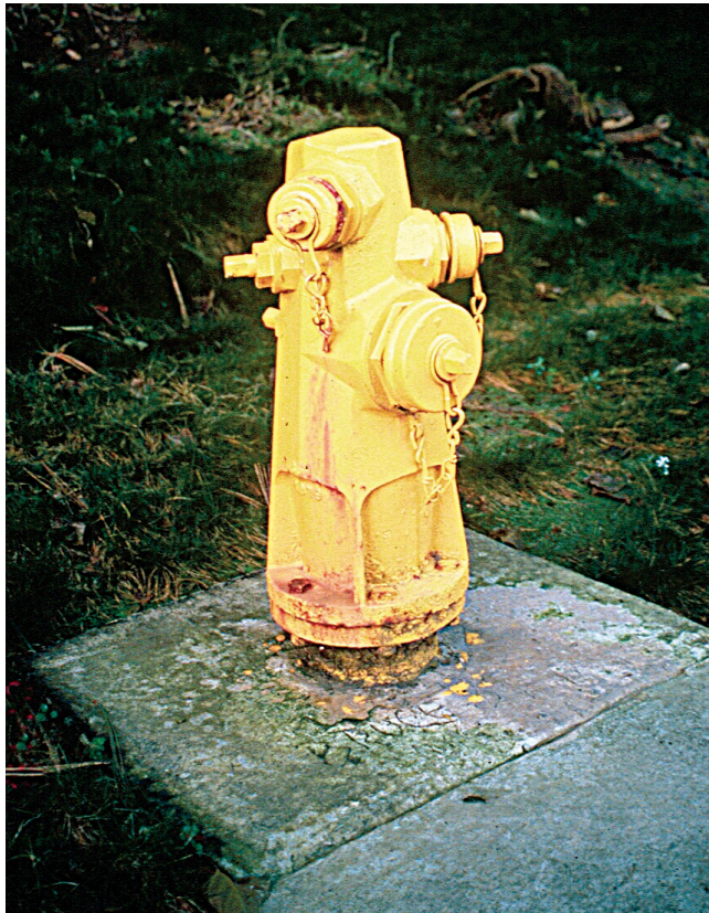
EXHIBIT 3 Wet Barrel Hydrant.
