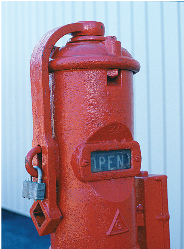
EXHIBIT 12 Post Indicator Valve (PIV).
