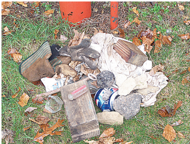
EXHIBIT 16 Debris Flushed Out of Underground Piping. (Courtesy of FM Global)
