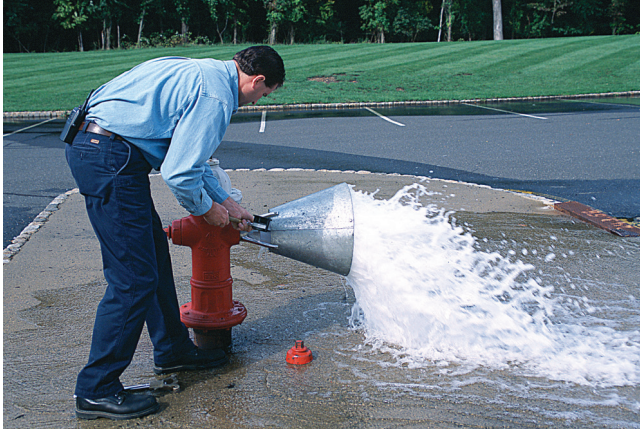
EXHIBIT 20 Flow Diffuser in Use During a Hydrant Flow Test.
