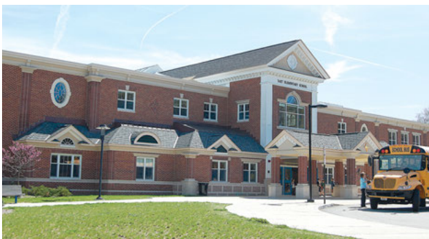
Exterior of an elementary school.
