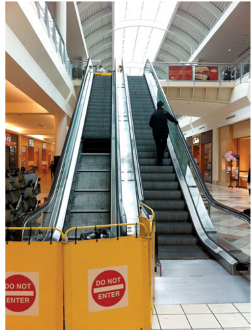
Escalator in a mall undergoing repairs.
