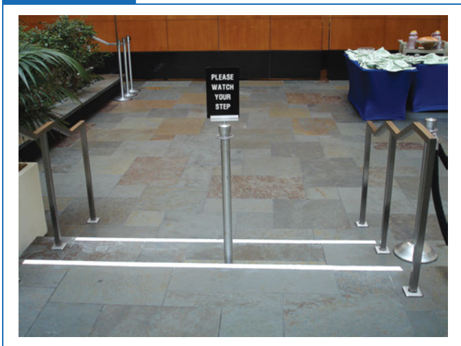
Egress route with small elevation difference in meeting room area. (Photo courtesy of Jake Pauls)
