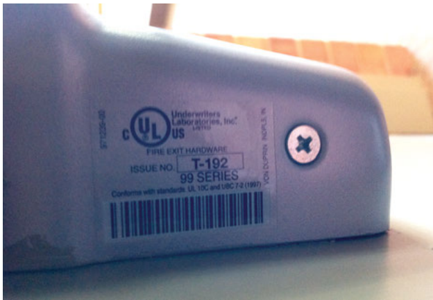
Fire exit hardware listing label.
