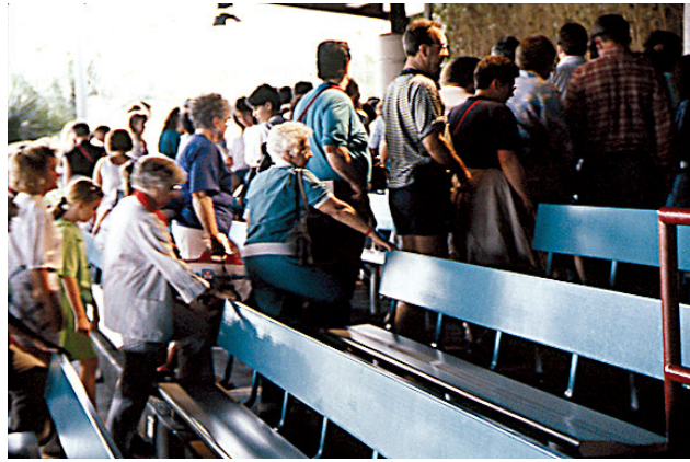
Bench seat backs used as handholds where handrails are not provided on aisle stair. (Photo courtesy of Jake Pauls)
