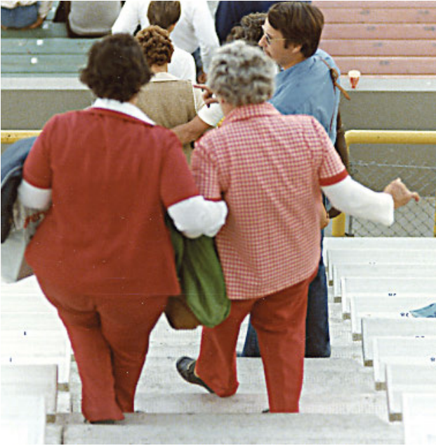
Cautious movement on grandstand/bleachers aisle stair without handrails. (Photo courtesy of Jake Pauls)
