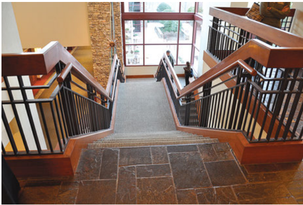
Guards and handrails. (Photo courtesy of Jake Pauls)
