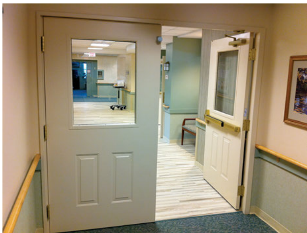
Cross-corridor smoke barrier doors, which are part of the “defend-in-place” protection strategy.
