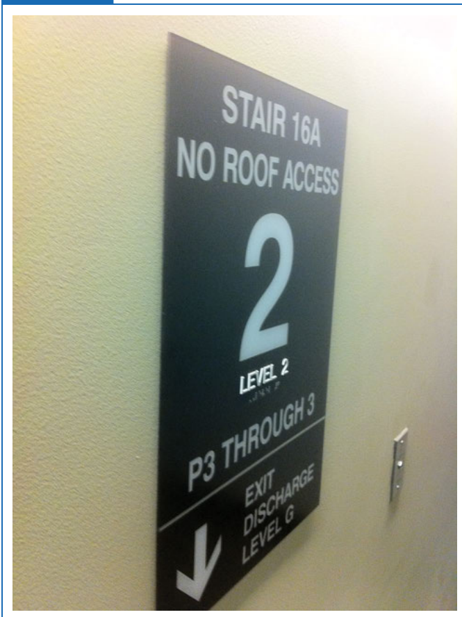
Stairway identification sign with tactile floor level designator.
