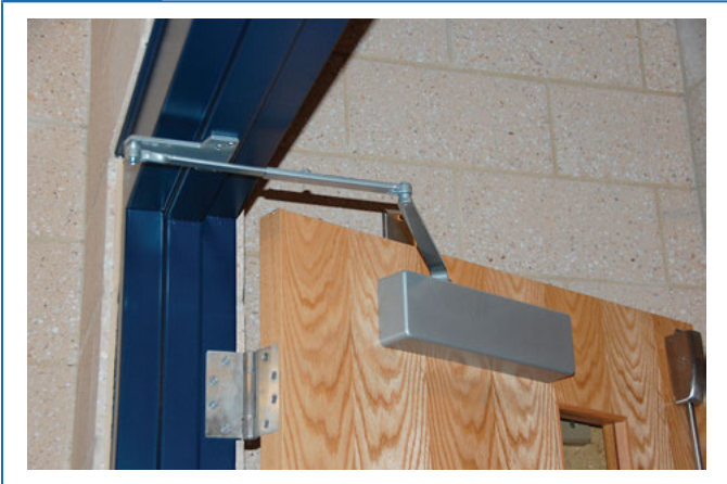
Door leaf with self-closing hardware.
