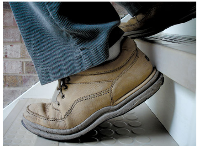
Tread nosing catches stair user’s heel. (Photo courtesy of Jake Pauls)
