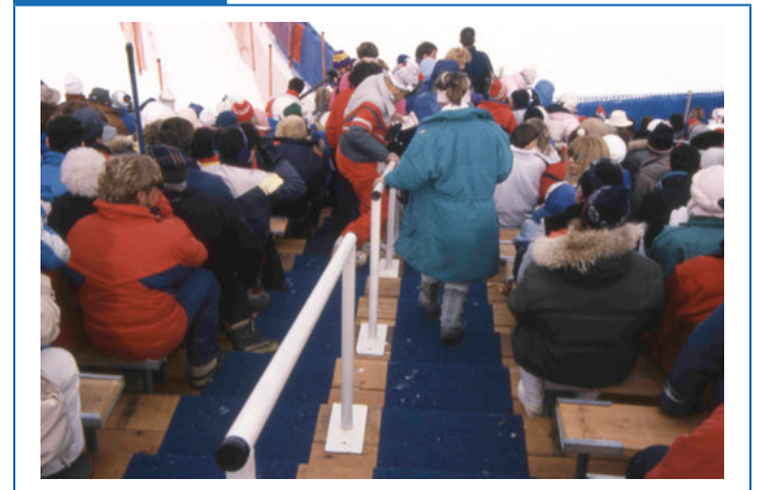
Intensive use of stadium aisle stair with center handrail. (Photo courtesy of Jake Pauls)
