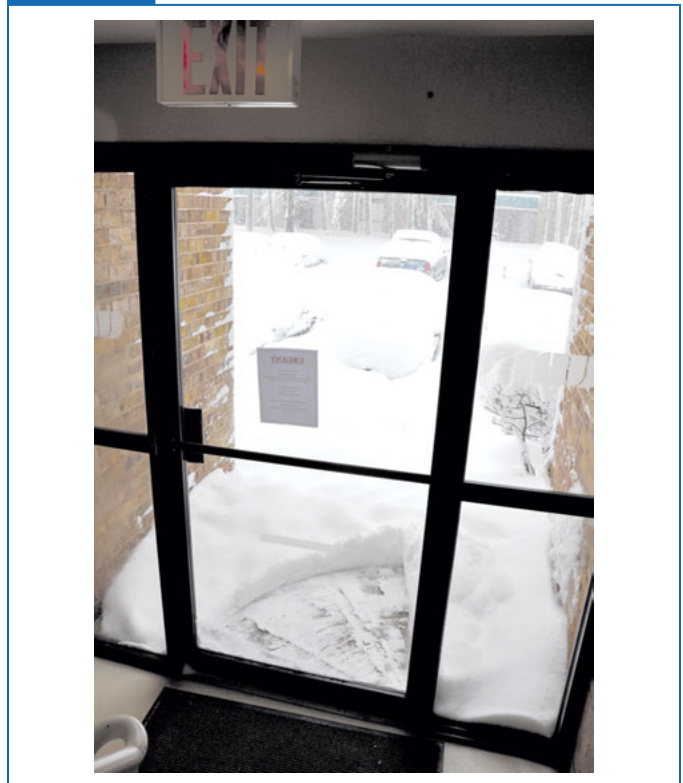
Snow accumulation pushed away by swinging the door open. (Photo courtesy of Jake Pauls)
