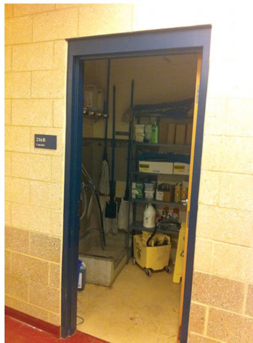
Janitor closet requiring protection.
