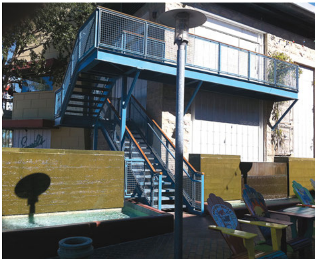
Guards at open side of exterior exit access balcony and stair.
