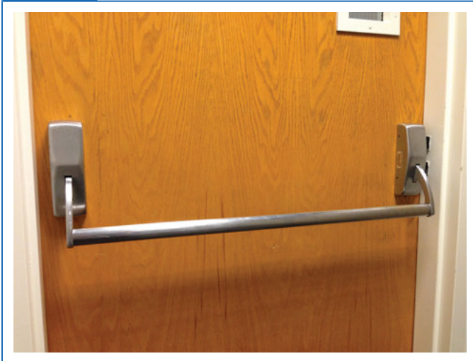
Latch release actuating member in the form of a bar.
