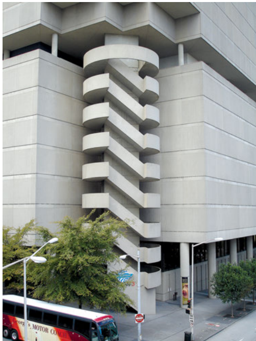
Outside stair with opaque visual barriers. (Photo courtesy of Jake Pauls)
