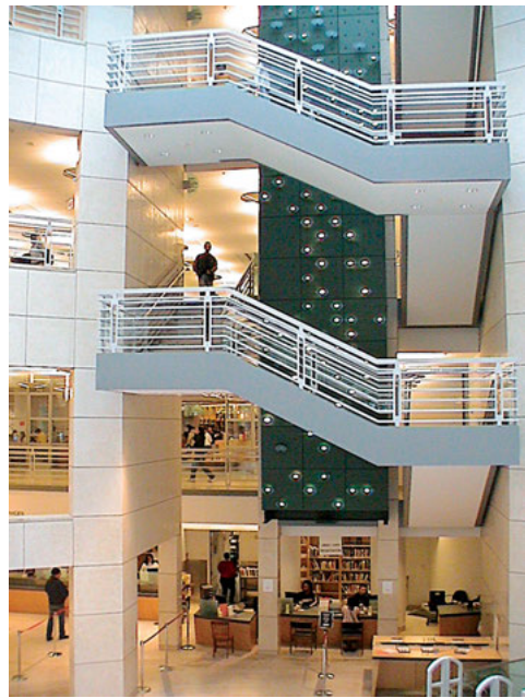
Vertical opening protected as an atrium in a library. (Photo courtesy of Jake Pauls)
