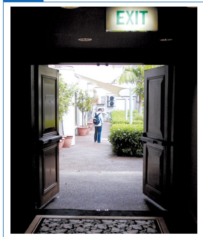
The three-part means of egress — exit access, exit, and exit discharge. (Photo courtesy of Jake Pauls)
