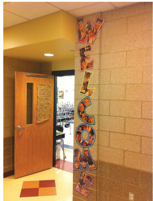
Classroom door swinging into recessed pocket in corridor.
