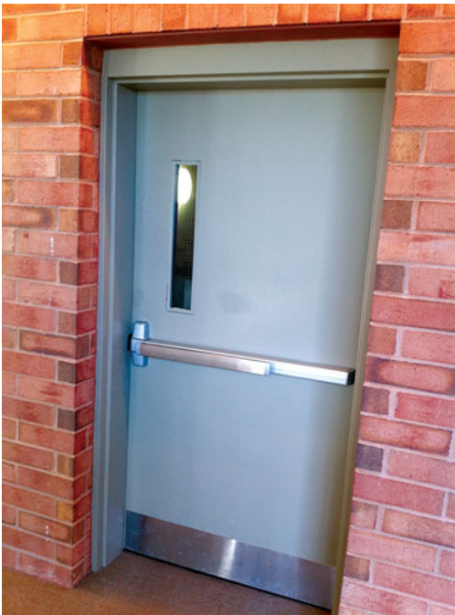
Fire exit hardware on fire-rated door.
