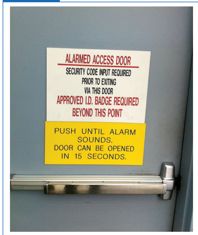
Door with delayed-egress hardware and conflicting information placards.
