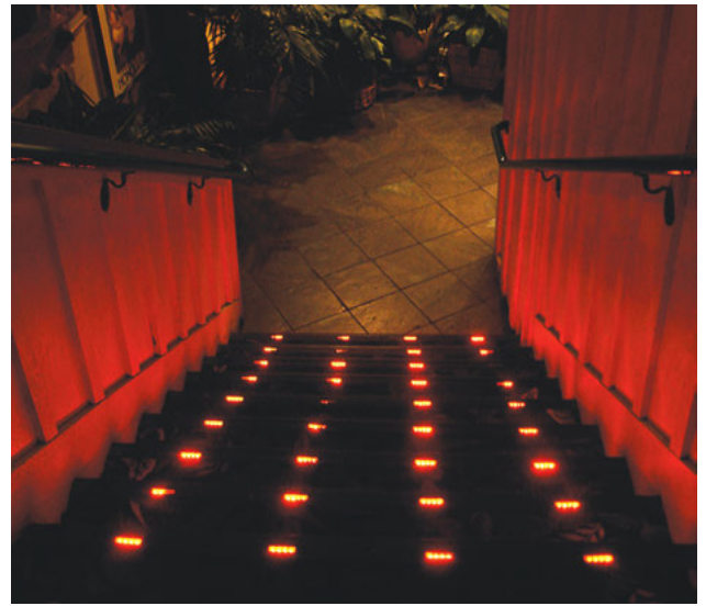
Interior stair illumination via lights at stair treads. (Photo courtesy of Jake Pauls)
