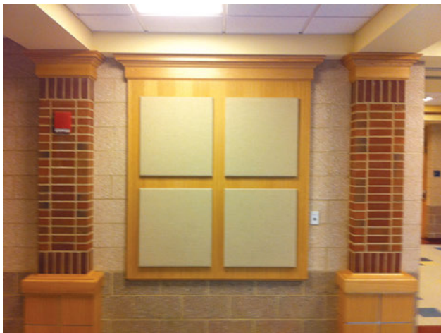
Acoustical panels constituting interior wall finish.
