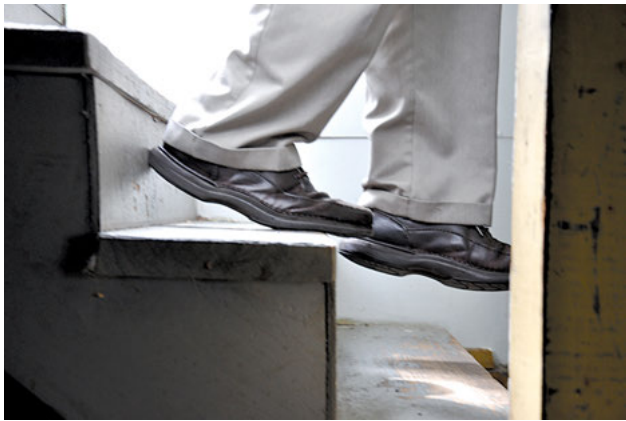
Stair user's toes extending over tread edge while heel scuffs riser. (Photo courtesy of Jake Pauls)
