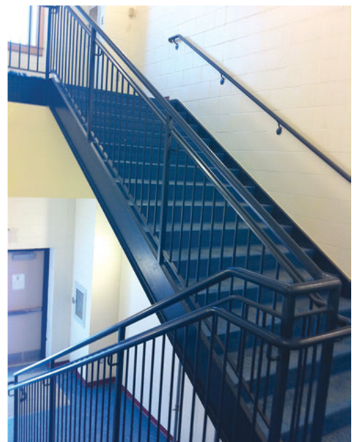
Stair with handrails and guards.
