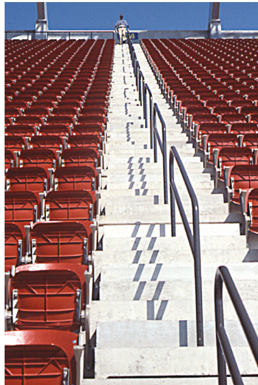
Center-aisle handrails with required gaps. (Photo courtesy of Jake Pauls)
