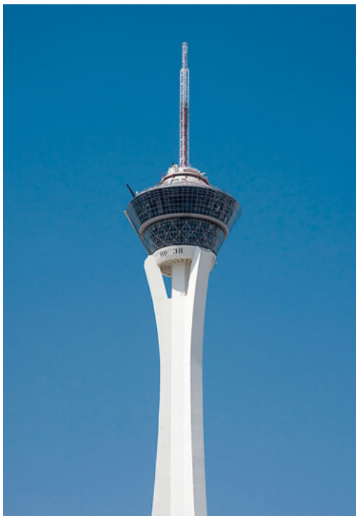
Stratosphere Tower, which employed performance-based design in its evacuation strategy. (© Julian Fletcher, Dreamstime.com)
