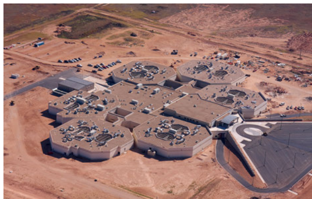
Detention facility aerial view with six distinct sleeping and living pods.
