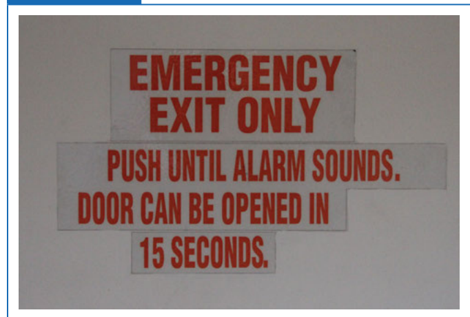
Signage on door with delayed-egress hardware.
