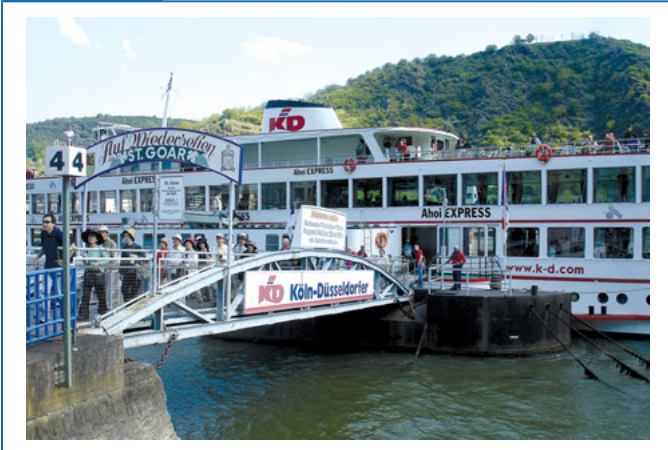
Vessel-boarding ramp subject to differing slope. (Photo courtesy of Jake Pauls)
