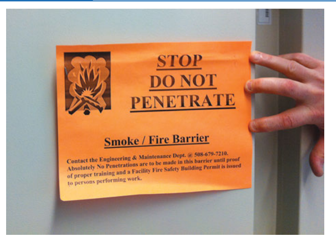
Placard with warning against penetration of smoke barrier.
