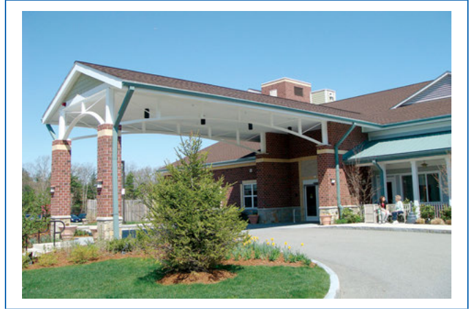
Main entrance of a nursing home.
