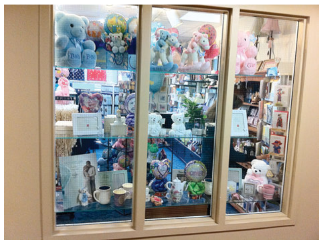
Large gift shop separated from corridor and protected as a hazardous area.
