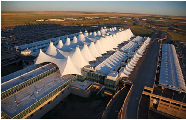
Example of a tensioned-membrane structure: Denver International Airport. (Photo courtesy of Denver International Airport)
