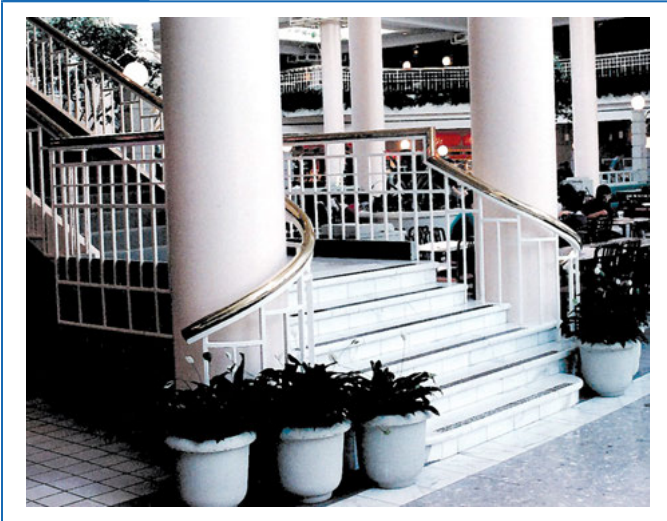
Potted plants prevent access to required handrails. (Photo courtesy of Jake Pauls)
