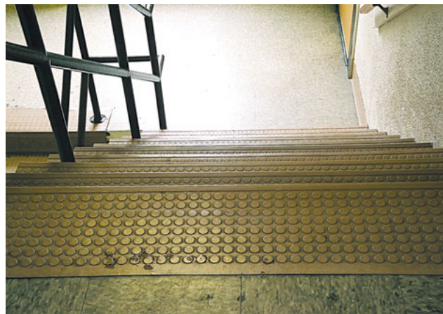
Nonuniformity in tread/riser dimensions identified by crouch and sight test. (Photo courtesy of Jake Pauls)
