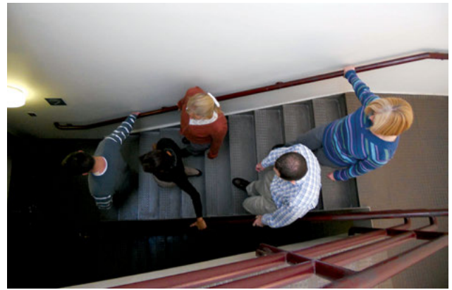
Overhead plan view of stair with handrails within maximum 30 in. (760 mm) reach.
