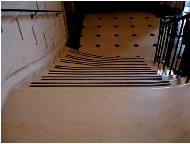
Tread depth variations on stair flight. (Photo courtesy of Jake Pauls)
