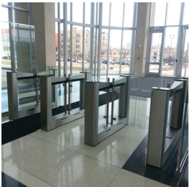
Security access turnstiles viewed from side providing egress. (Photo courtesy of U.S. General Services Administration)
