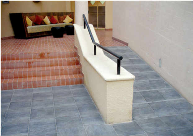
Ramp at side of stair. (Photo courtesy of Jake Pauls)
