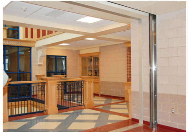
Track system and door stop for sliding door to isolate vertical opening.
