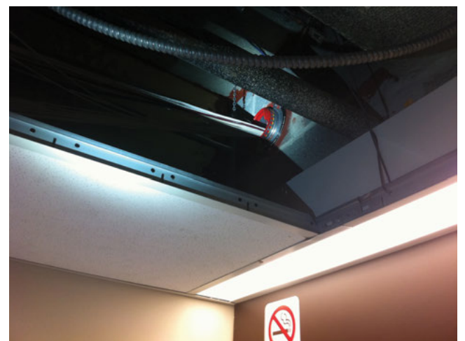
Above-ceiling space at a smoke barrier in a hospital.
