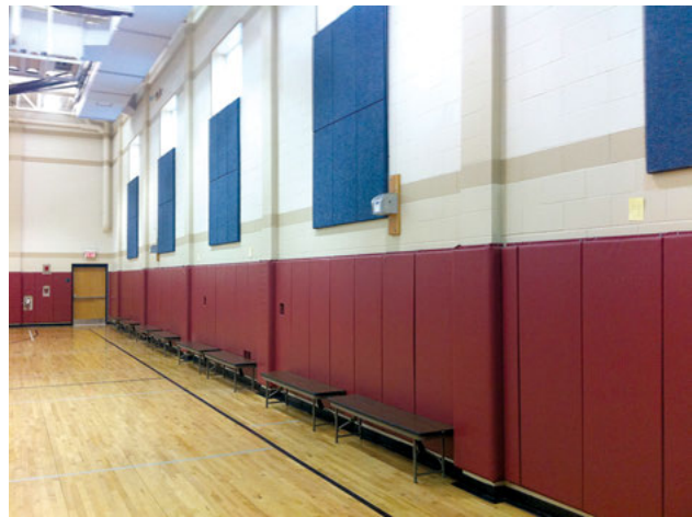
Protective padding and acoustical panels constituting interior wall finish.
