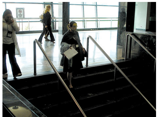
Poorly lighted interior stair near brightly lit window space. (Photo courtesy of Jake Pauls)
