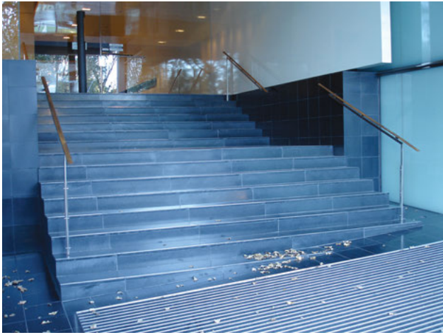
Stair risers adjoining a sloping walk.
