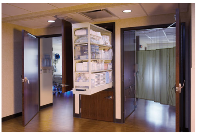
Nurse server, or sliding supply shelving unit, in corridor wall.
