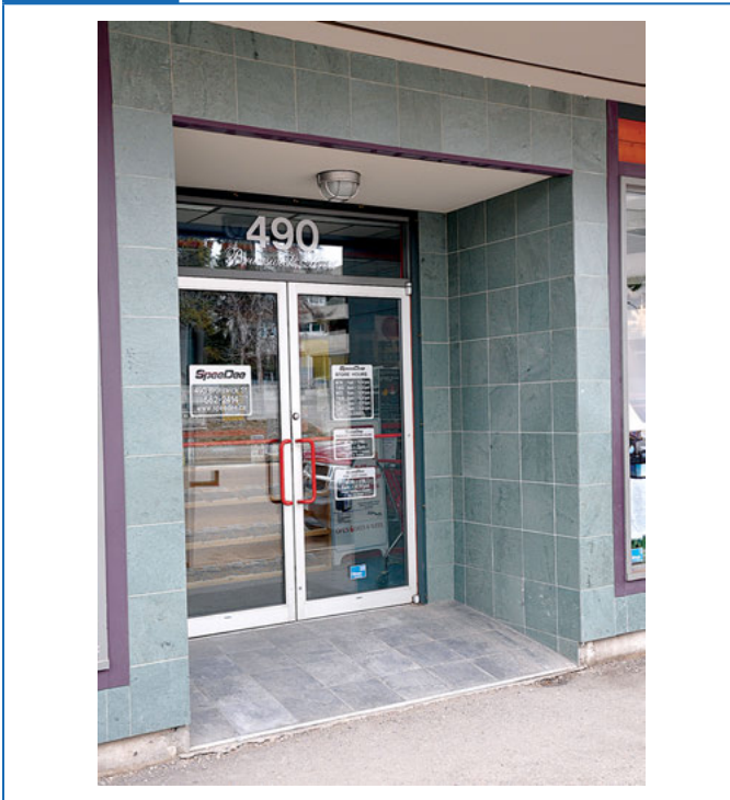
Ramp at front door that permits accessible route to continue to public way. (Photo courtesy of Jake Pauls)
