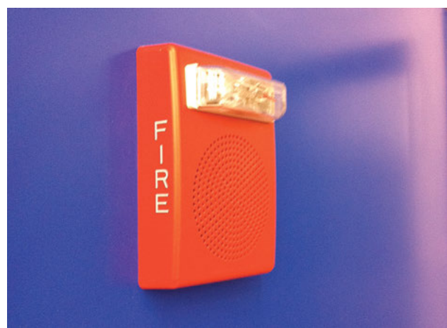
Alarm system appliance to provide visible signal and initial audible alerting tone to occupants.
