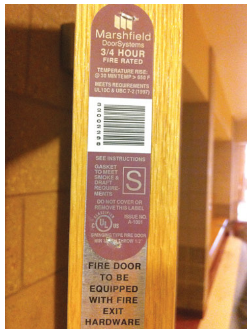
Listing label affixed to door leaf of a fire door assembly.
