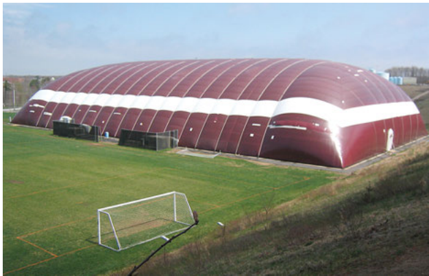
Example of an air-inflated structure: the former Plymouth Sports Dome, Plymouth, Massachusetts.
