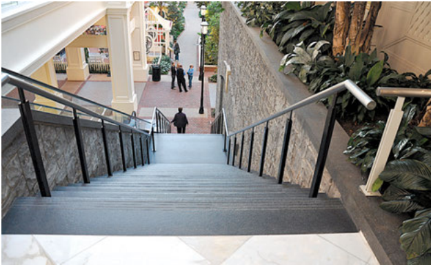
Existing stair width that does not require intermediate handrail. (Photo courtesy of Jake Pauls)
