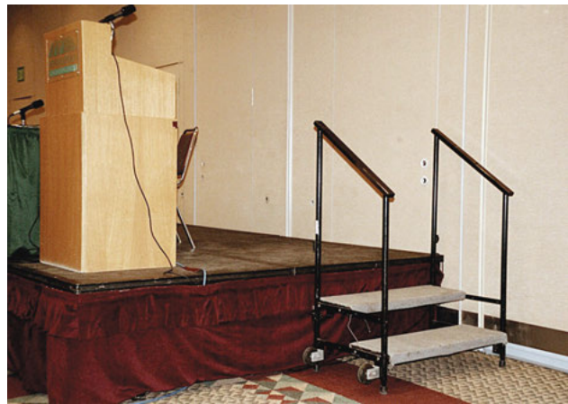
Platform stair with handrails. (Photo courtesy of Jake Pauls)
