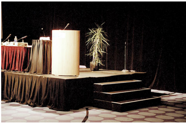
Platform stair without handrails. (Photo courtesy of Jake Pauls)
