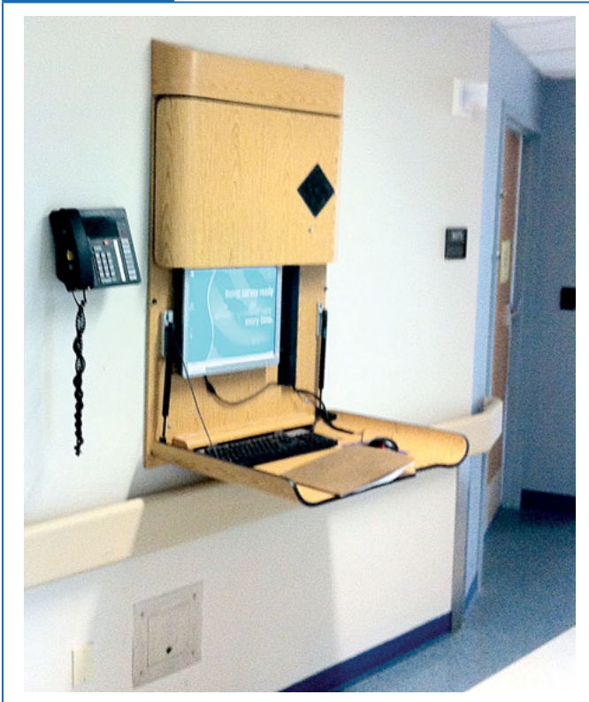
Corridor width projection created by charting station.
