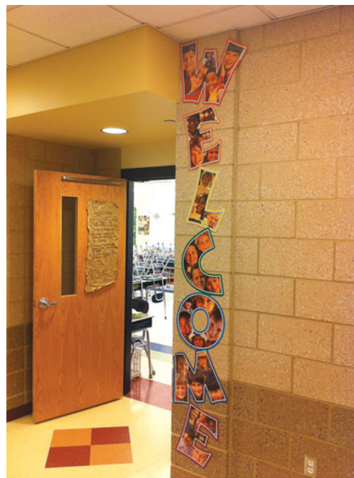
Door set into recess in corridor wall.
