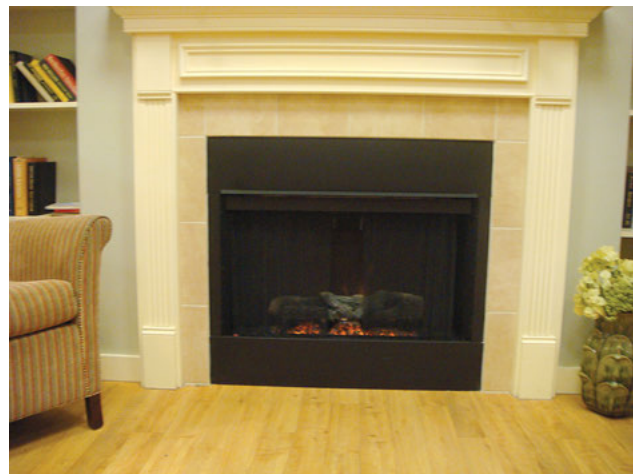
Gas fireplace in nursing home resident lounge space.
