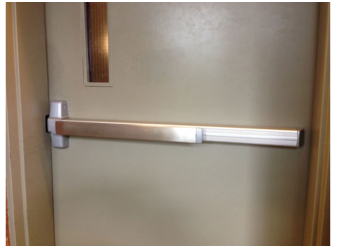
Latch release actuating member in the form of a push pad.
