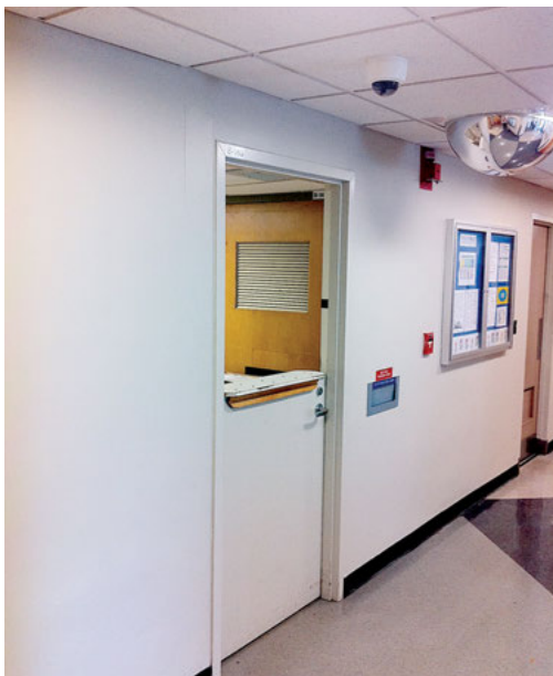
Dutch door in corridor wall.
