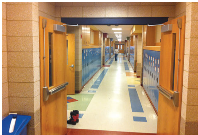
Corridor with minimal encroachment.
