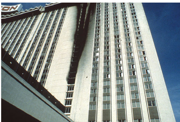
Resulting fire spread involving elevator lobbies on eighth through twenty-fourth floors.
