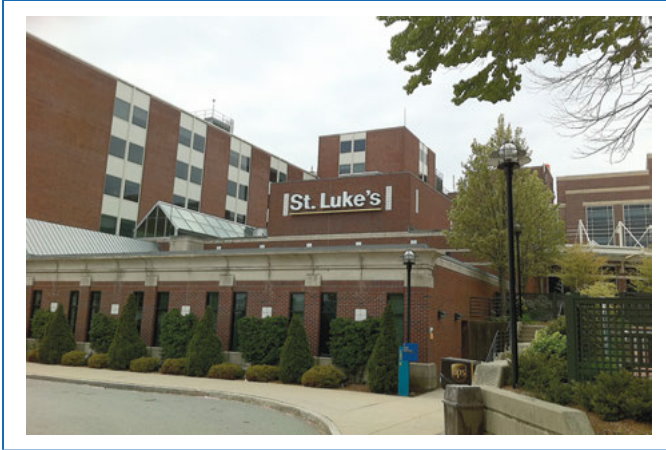
Main entrance of a hospital.
