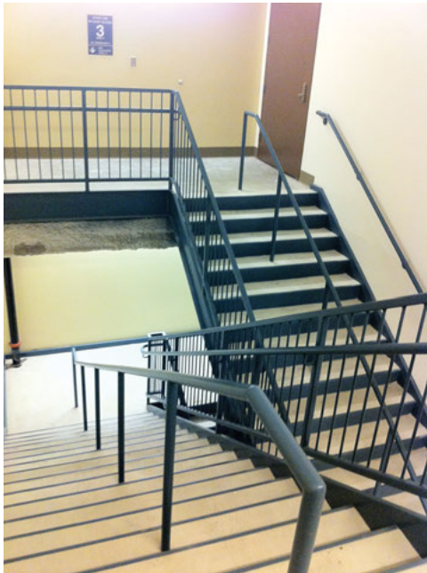
Enclosed exit stair with intermediate handrails.
