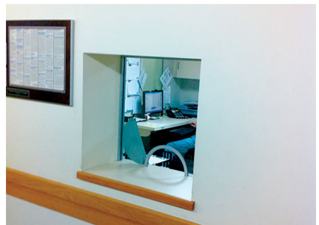
Pass-through opening in window in corridor wall.
