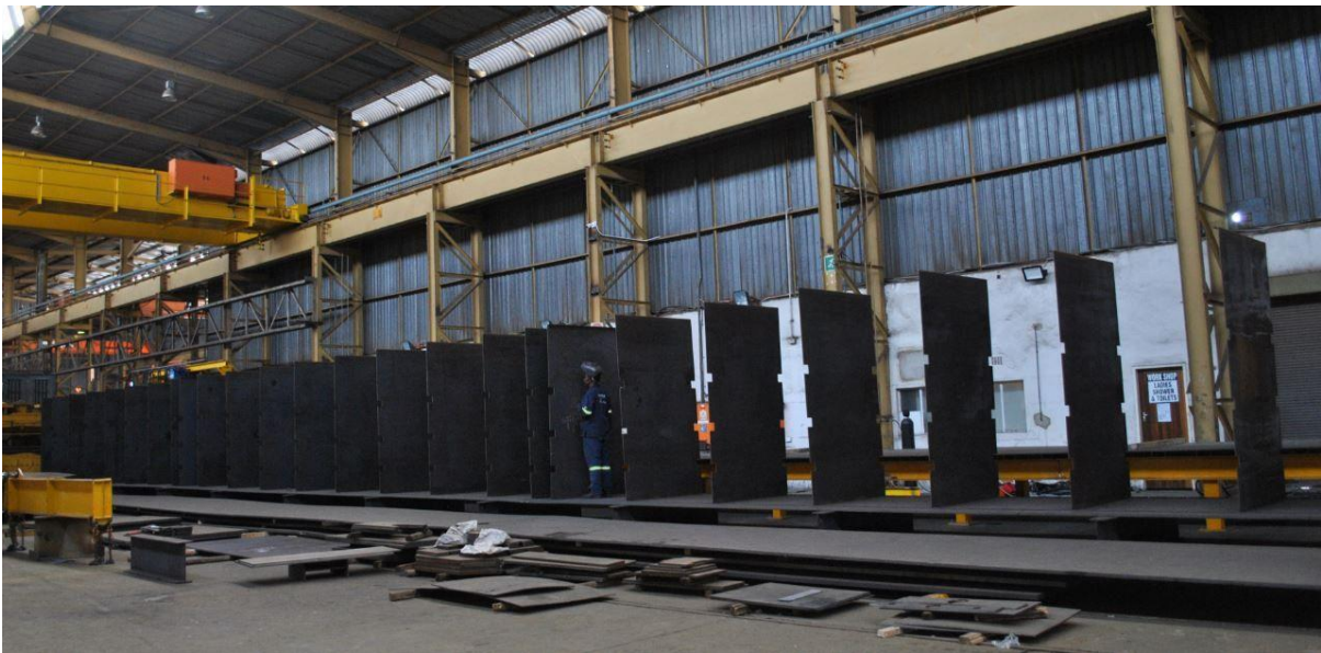
Construction of a Bridge Crane – Baffle Plates Exposed
